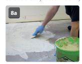
Starting with a few square meters at a time apply Mapei Ultrabond ECO 380 to the substrate using a 2mm (A2) tooth comb spreader (8a). Do not use Mapei Ultrabond ECO 380 as a filler to level out gaps, cracks or uneven substrates as this will greatly reduce the coverage achieved and increase drying times, plus effecting the ability to **bond properly**. Any uneven screed or concrete floors should be levelled with a renovation screed first. Mapei recommend Ultraplan Renovation Screed for this.
