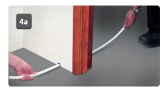
When floor heating pipes need to pass through walls, drill the holes before laying and fixing boards to prevent any damage to the boards. Protect and seal the pipe ends with tape. To prevent kinking, one person should feed the pipe through the hole whilst another draws the pipe through from the other side, it is a good idea to use pipe conduit to run through walls (4a).
